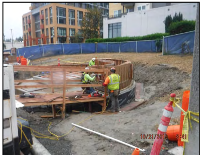
Mid-Tunnel Shaft stair case and top lid rebar and form
