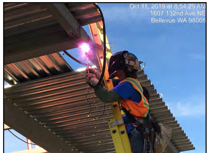
Welding the south-side station platform canopy to the columns, looking southwest.
