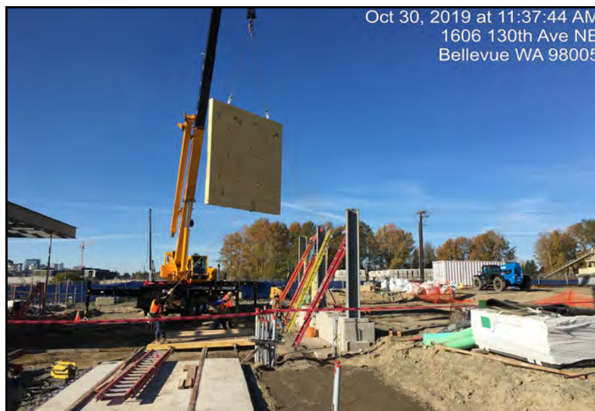
E340 Bel-Red: Placing pre-cast panels at Bel-Red/130th Ave Station.
