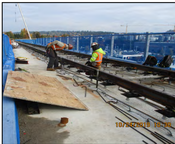
Plinth Rebar installation at Wilburton Station. (Area 4)
