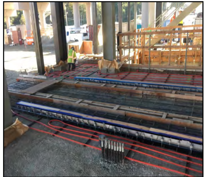
Floor Slab Preparation—OMF
