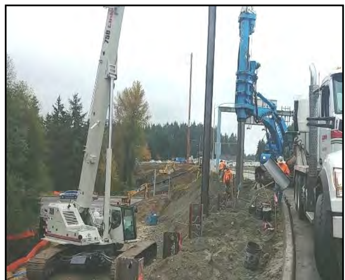
Placing piles for support of excavation in Work Area 4.
