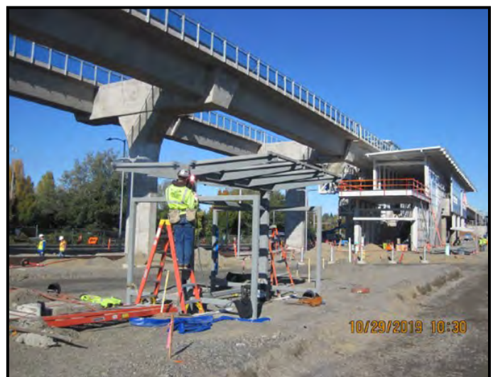
Welding transit shelter awning steel beneath the guideway.
