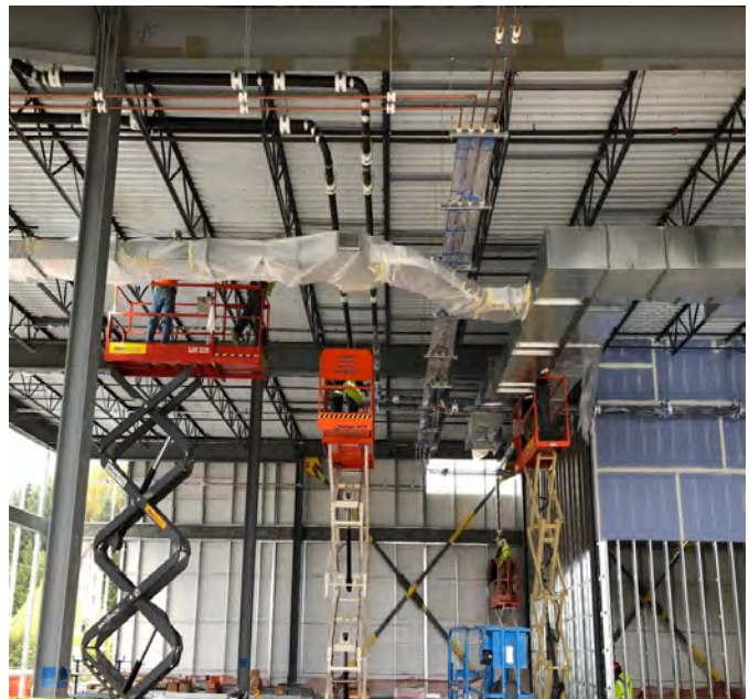
OMFE—HVAC duct installation on the 2nd floor.
