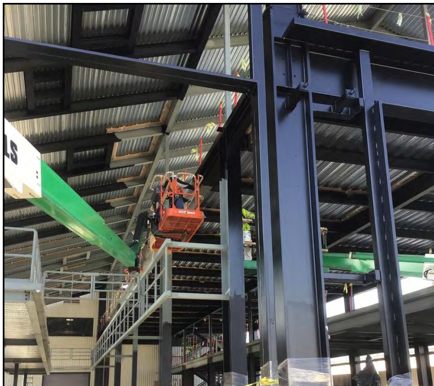
OMF– Ongoing painting
