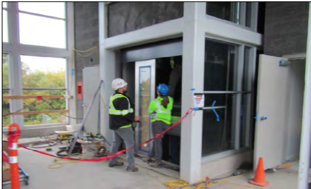
N160 – Installing sliding glass doors for elevator.
